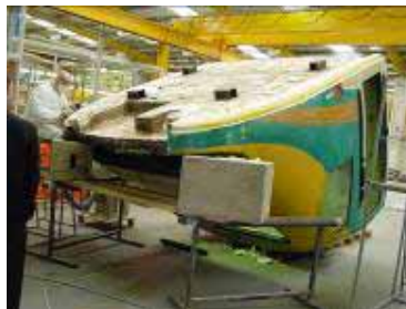
A composite high speed train cab undergoing structural repair
